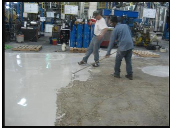
From the mix station, the Agri-Rok was poured onto the floor. One man screeds the material to approximately  $\frac{1}{4}$ " using a gage rake. After gaging, the material was smoothed using a magic trowel (a squeegee or hand trowel could also be used).
